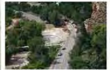
MILEPOST 85.43 - Aerial view of damaged eastbound lane but passable westbound lane near Big Thompson Elementary School. Loss of embankment and pavement.
