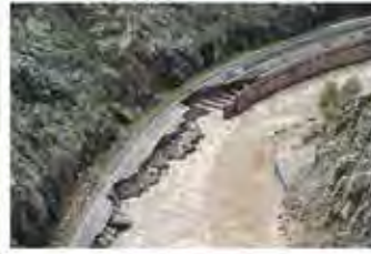
MILEPOST 82.6 - Upstream view of a significantly damaged road along the Big Thompson River near Dickson Gulch, with a large portion of the road washed out. Reflects undermined/loss of retaining wall backfill, pavement, and riprap embankment; exposure of wall tie backs and bedrock.
