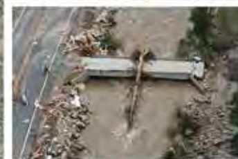
MILEPOST 65.83 - Aerial View of Rock Canyon Rd access bridge. Bridge approaches are undermined with large debris piles at bridge and on US 34.
