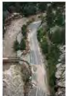
MILEPOST 68.27 - Aerial view of highway overtopping with sediment and debris accumulation on US 34 near Noels Draw.
