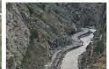
MILEPOST 83.0 - Aerial view through the "Narrows" portion of the Canyon shows heavy highway damage and frequent instances of overtopping with debris fields.
