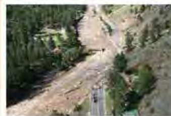
MILEPOST 76.45 - Aerial view of US 34 completely washed out at Rose Hall Way. Loss of access bridges at Rose Hall and Moodle (west of Rose Hall) isolated residents on the south side of the highway. The flooding also caused extensive property damage within this reach.
